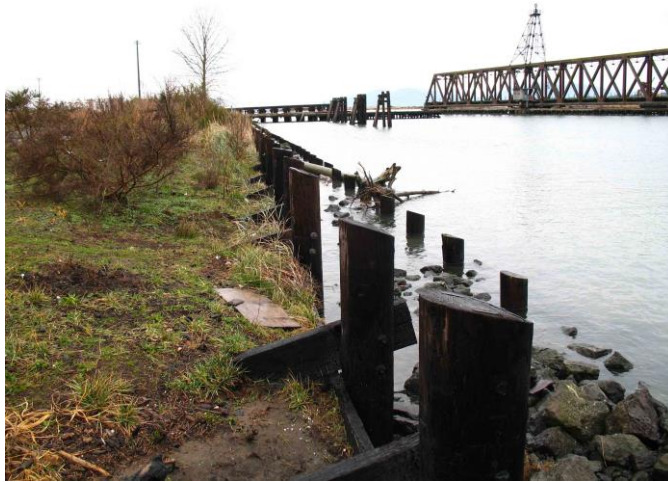
Figure 3. Creosote timber bulkhead
