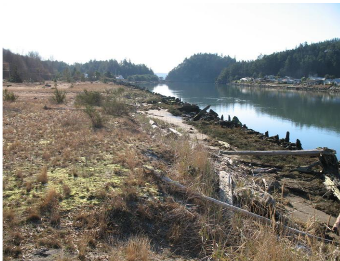
Figure 22. Deteriorated creosote treated bulkhead
