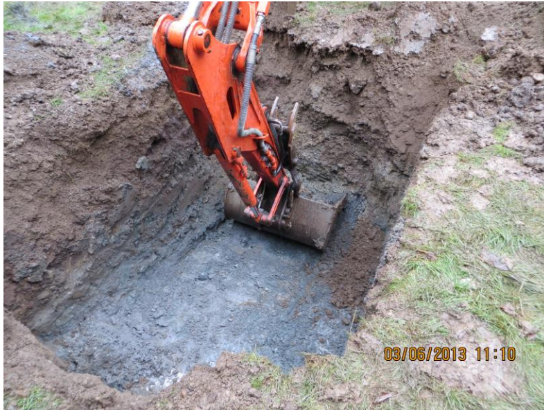
Figure 29. Abandoned heating oil tank remediation (Kukutali residence)
