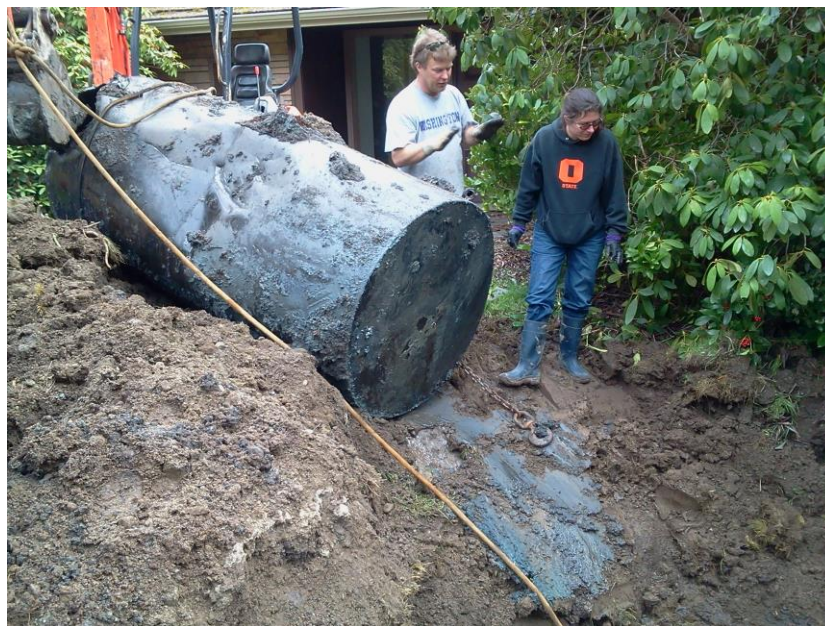
Figure 30. One of three leaking heating oil tanks removed from Kukutali residence site
